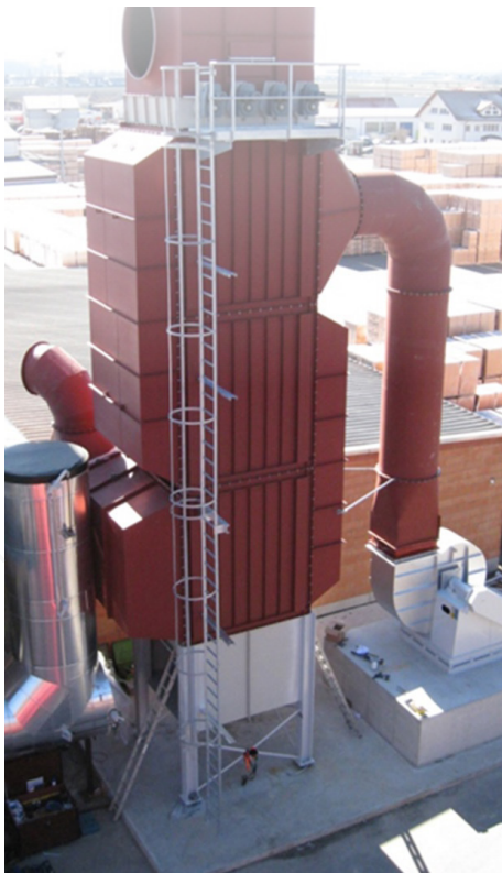
Flue gas heat exchanger
