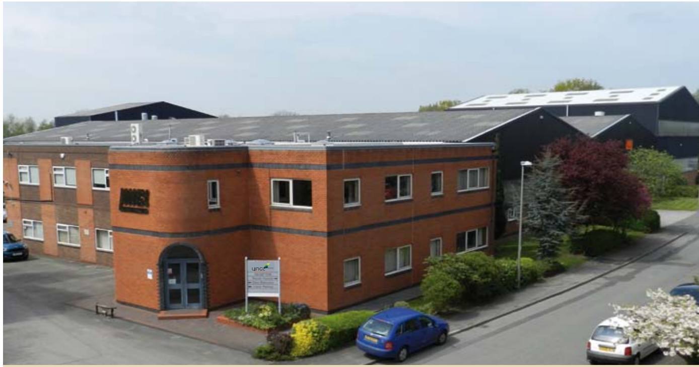
Aerial View of LINGL LUK Premises
