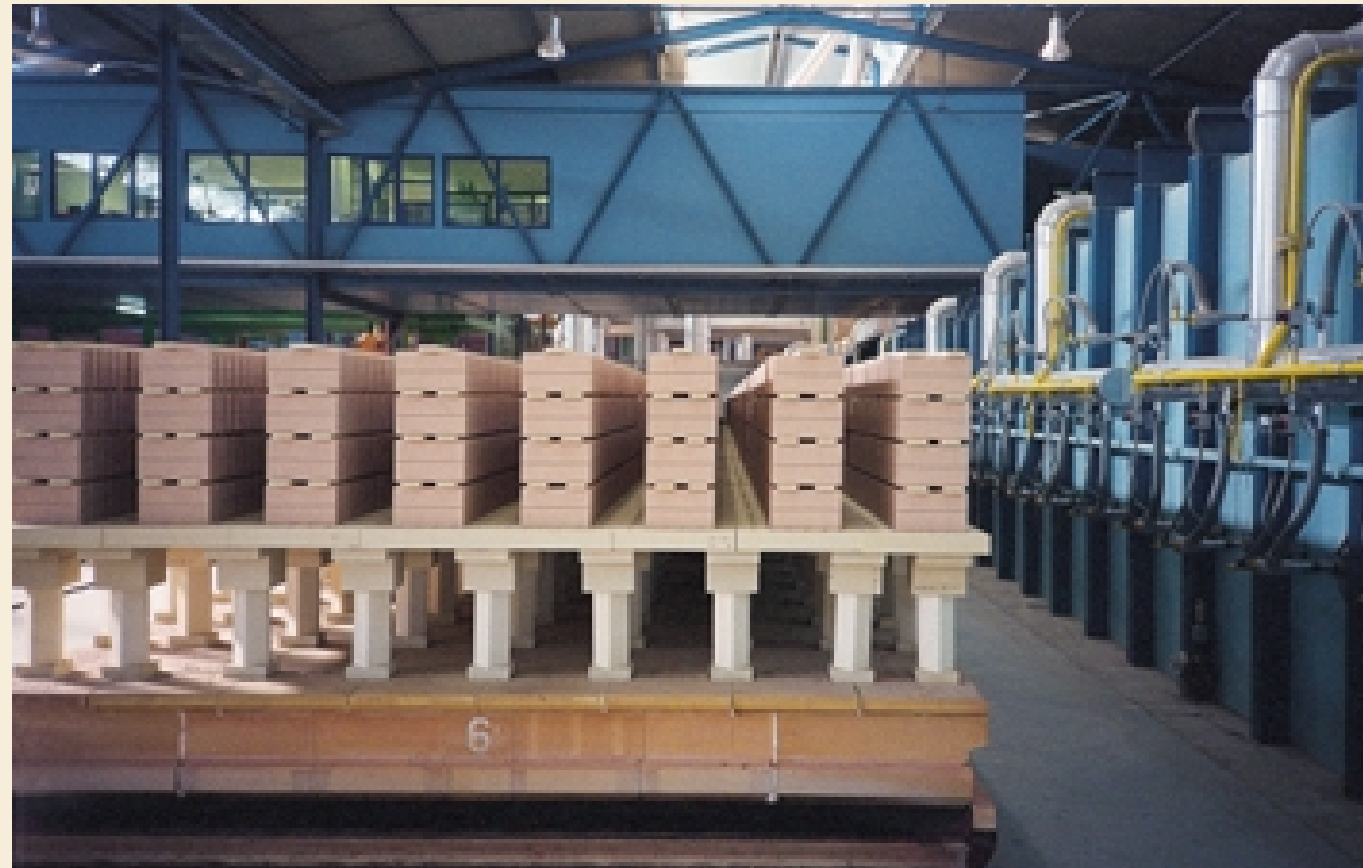
▼ Tunnel kiln cars with skirting strips, Lingl tunnel kiln with side firing facility
