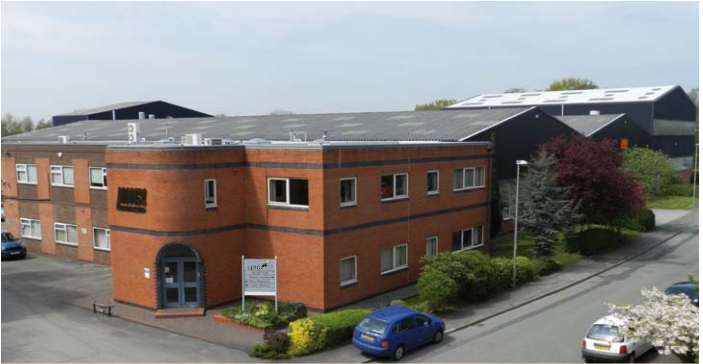
Aerial View of Lingl LUK Premises
