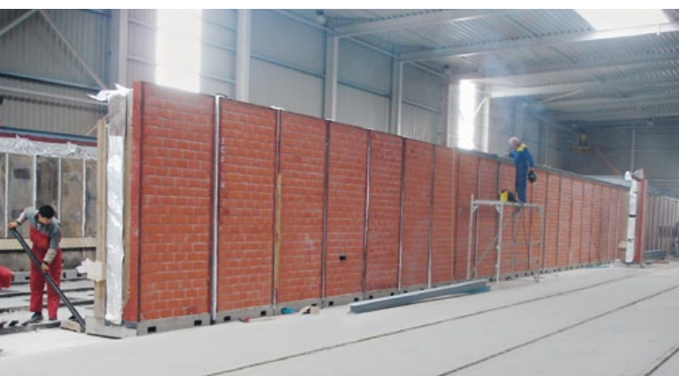
Modular kiln – assembly of wall modules Four modulaire – pose des modules de mur
