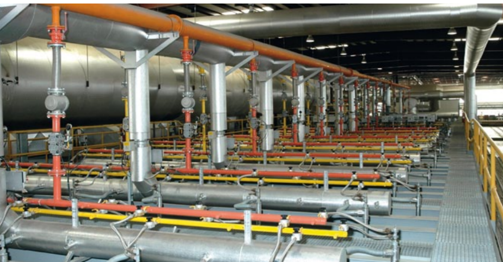
Dual fuel firing system for landfill gas and natural gas Installation de chauffage double à biogaz et gaz naturel
